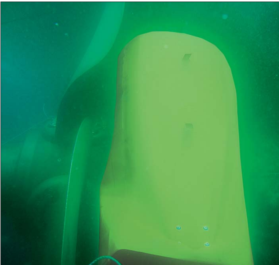
The Hydrex flexible mobdocks allow Hydrex divers to perform permanent underwater stern tube seal repairs.
