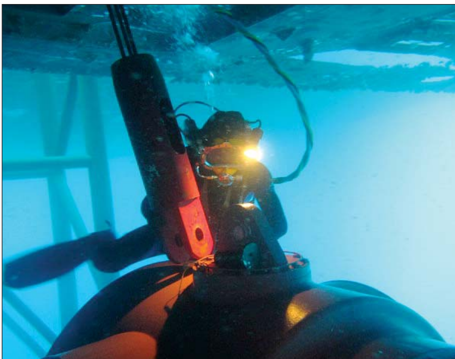
Hydrex diver/technician during reinstallation of azimuth thruster unit.
