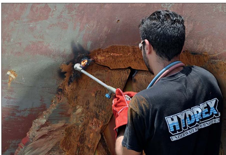
Hydrex technician making a crack arrest.
