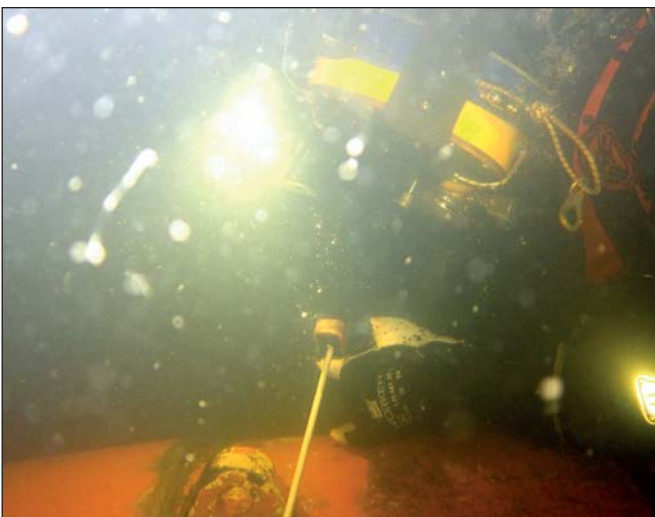
Diver/technician performing welding work on rope guard in Antwerp.
