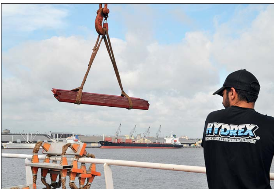
Stiffeners were then lowered and installed on the doubler plate.
