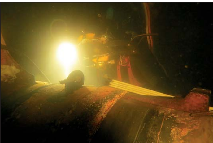
Diver/technician reinstalling the rope guard.
