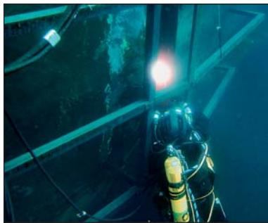
**H**ydrex on-site hull repair services include the renewal of both small and large areas of damaged hull plating. These repairs can be carried out above or below water, according to the circumstances, with tailor-made mobdocks. Normal commercial activities can therefore continue without disruption. These operations follow the Hydrex procedure for welding cracks in the vessel's shell plating and they are approved by the major classification societies.
