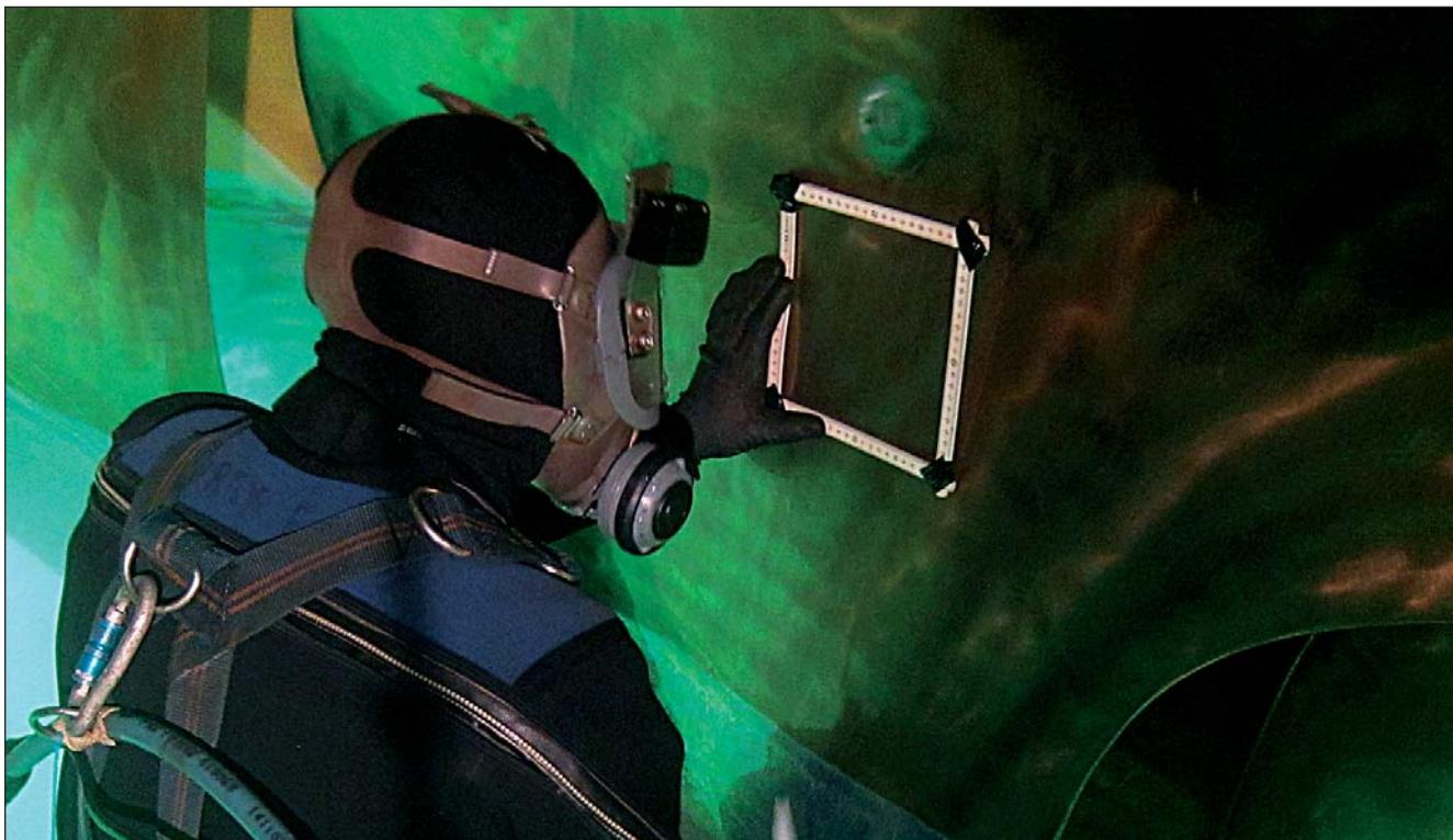
Over the years the Hydrex R&D department has continuously improved underwater repair techniques to make it possible for Hydrex diver/technicians to perform permanent repairs on seals, thrusters, rudders and almost any other part of the underwater vessel without the ship needing to go to dry-dock.
