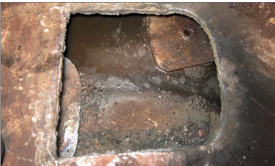
The damaged area was cut away.
