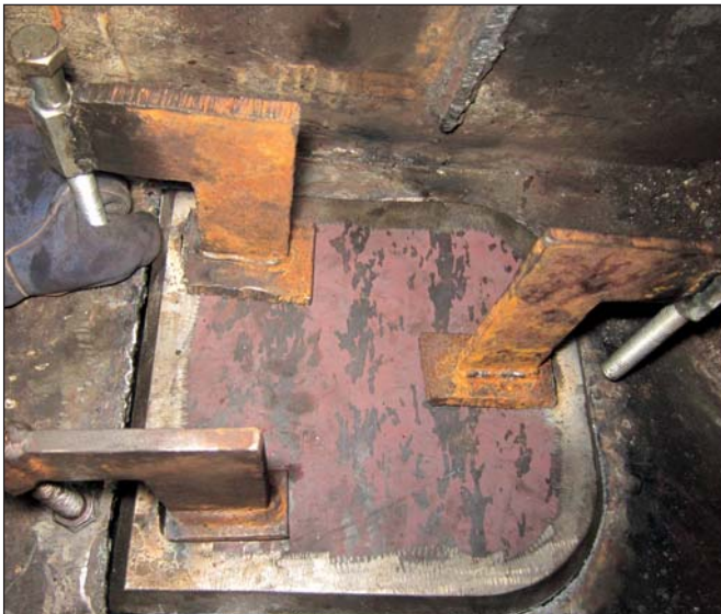
A new insert plate measuring 300 x 300 mm was positioned.
