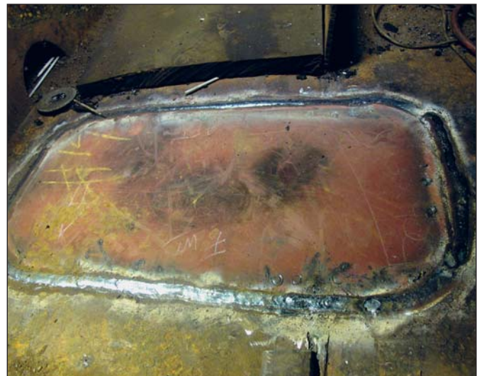
New insert repair after full penetration weld.
