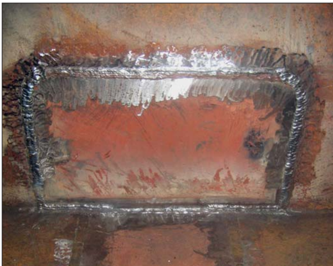
Framework reinstalled over new insert plate.
