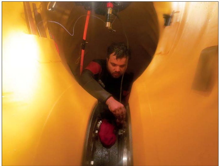
Inside the stern tube seal flexible mobdock divers can work in drydock-like conditions.
