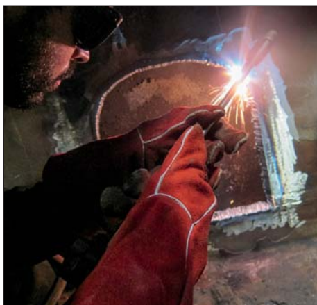
Opening in plate prepared inside tank.
