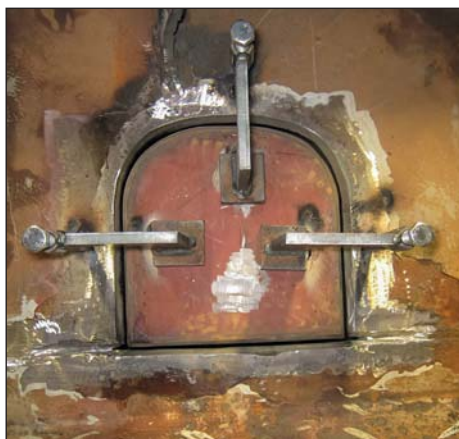
Insert cut and fitted.
