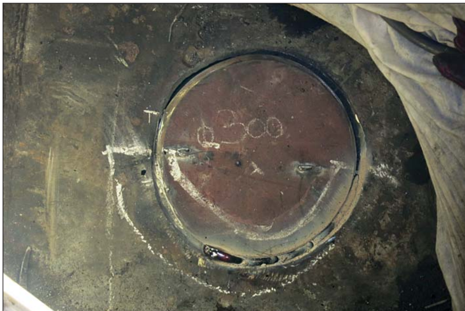
New insert positioned and secured.
