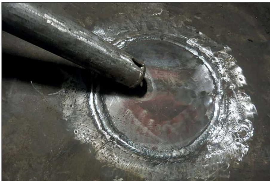
Fully welded insert.
