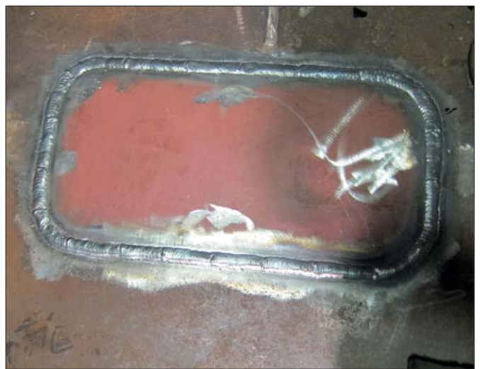
Fully welded insert plate.
