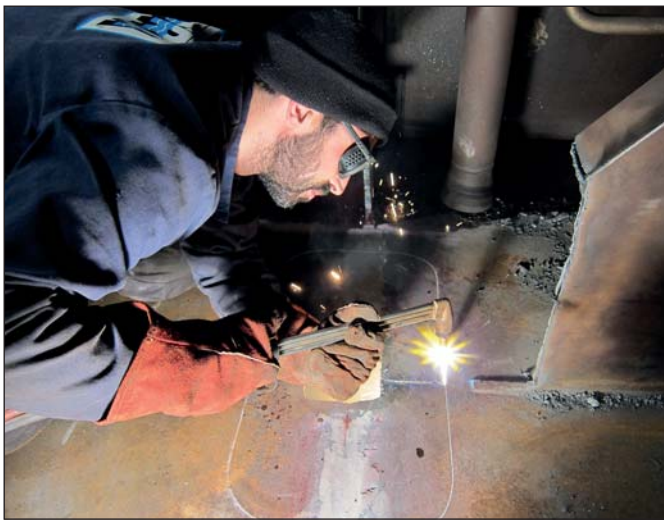
Cutting away the required area around the crack.
