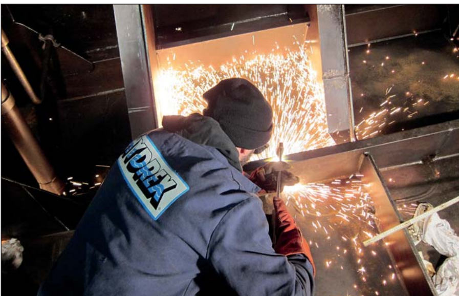
Removal of the frame covering the damage.
