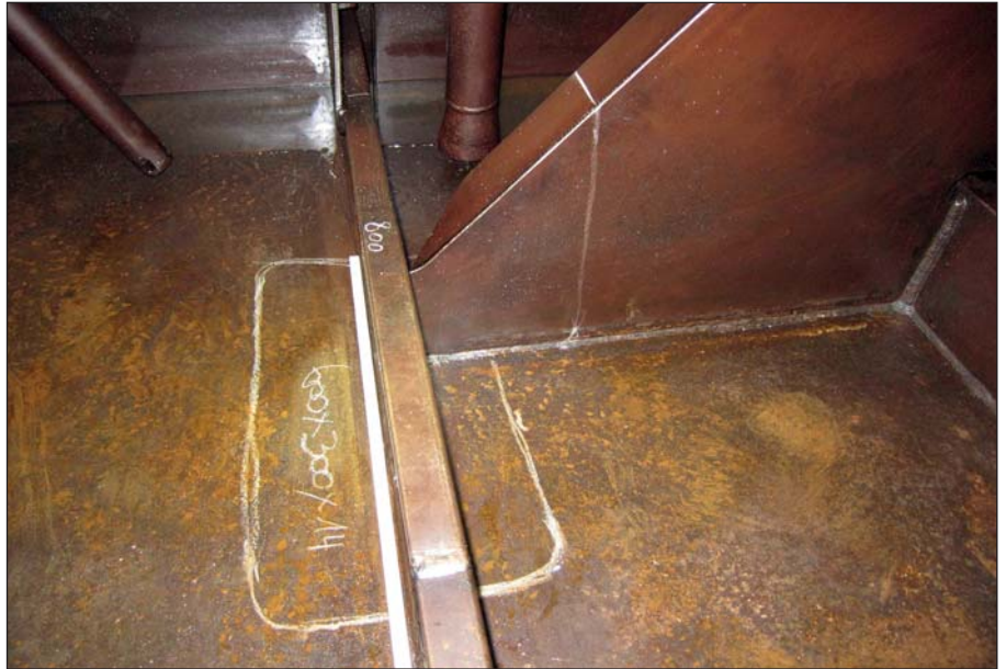
The plating and frames that needed to be removed were first marked.
