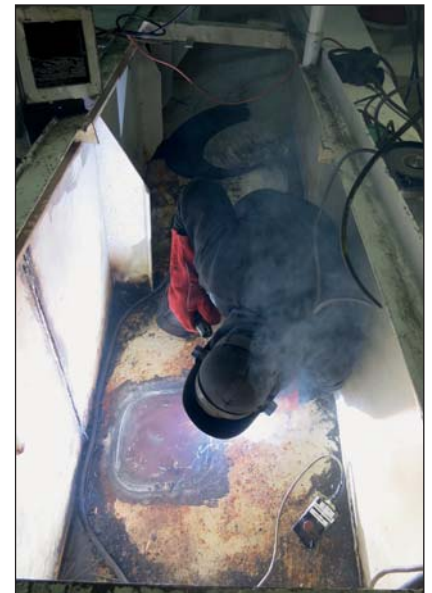
Securing new insert plate in Antwerp.
