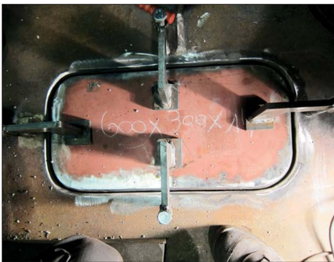
Fitting of the new insert.
