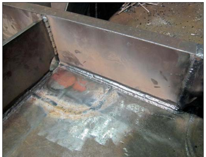
Reinstalled frame covering the new insert.
