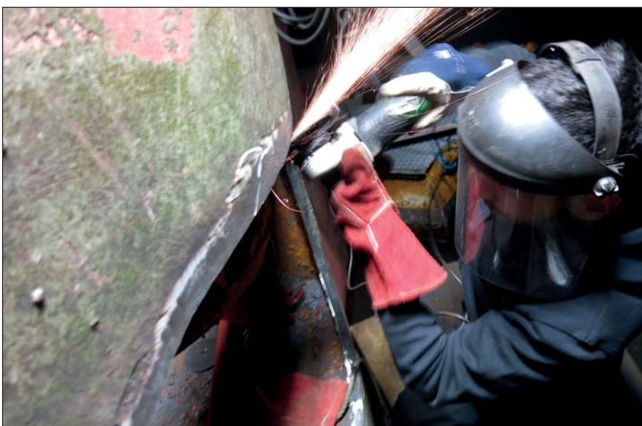
Beveling the edge of the rudder plate to fit the new cover plate.
