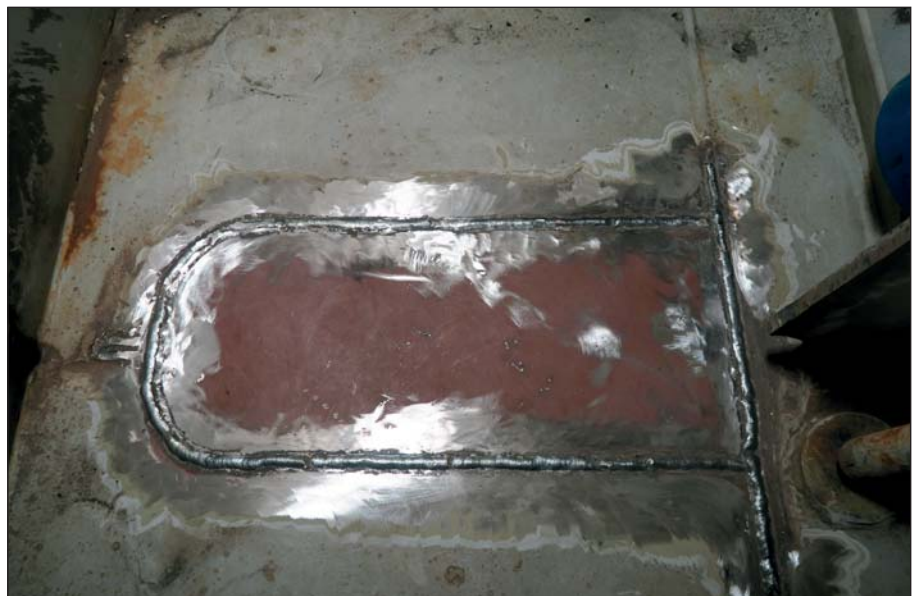
Insert after full penetration weld.
