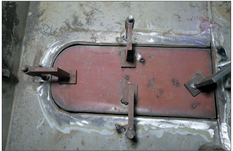
New insert positioned and secured.
