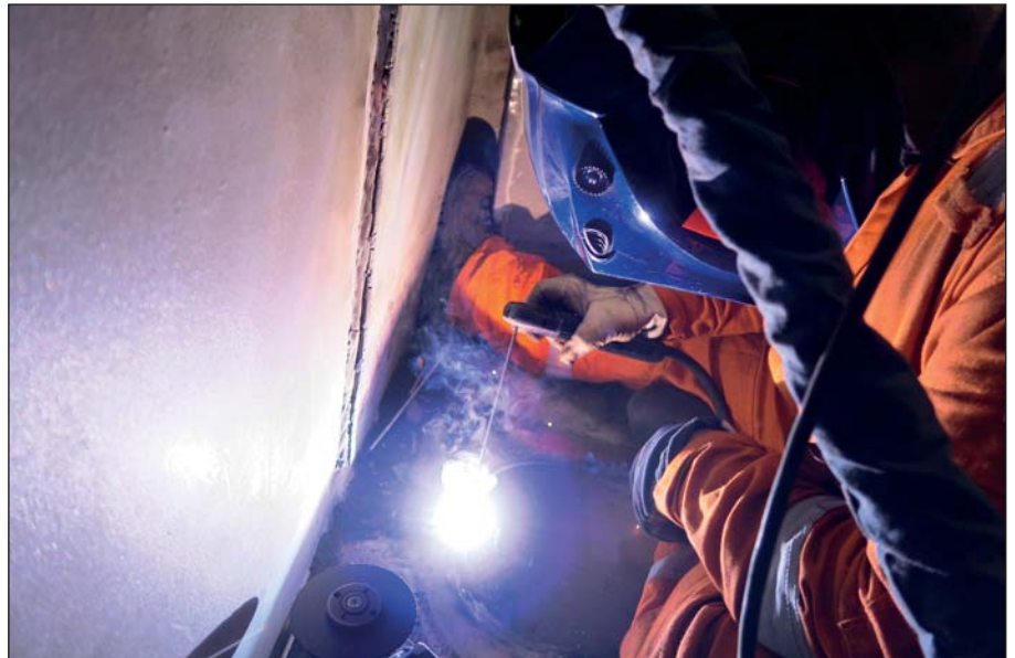
Welding the insert.
