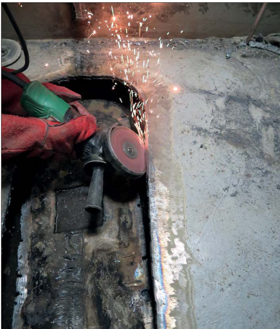
Preparing the edges of the area for the insert.
