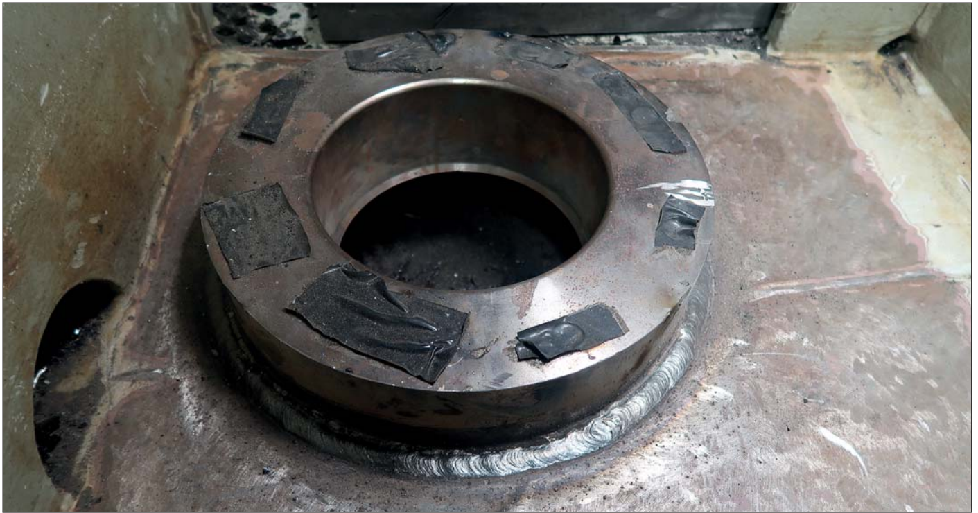
The base valve of the new system was positioned and secured with a full penetration weld.
