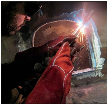
Opening in plate prepared inside tank.
