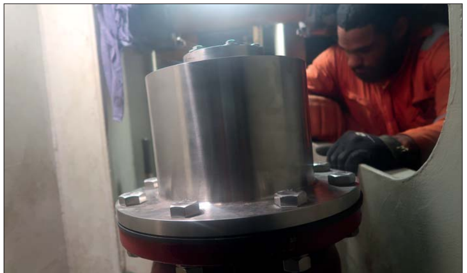
After the NDT test the valve was installed on top of the flange.
