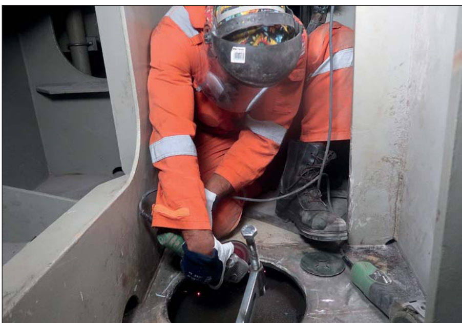
Preparing the edges of the hole.
