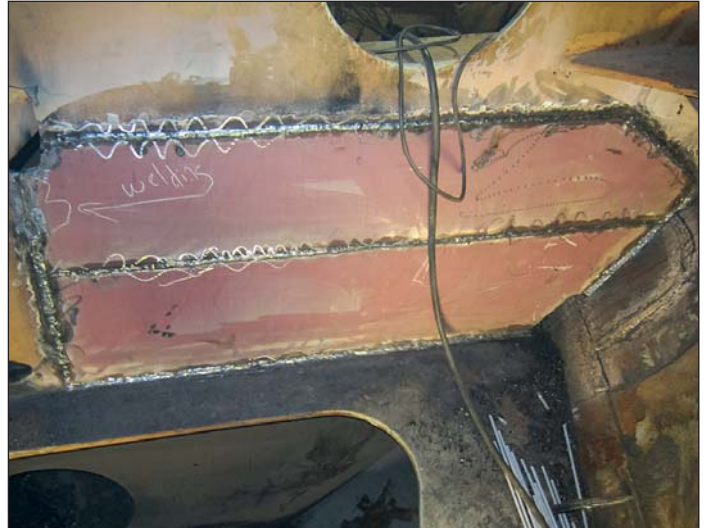
New frames welded.
