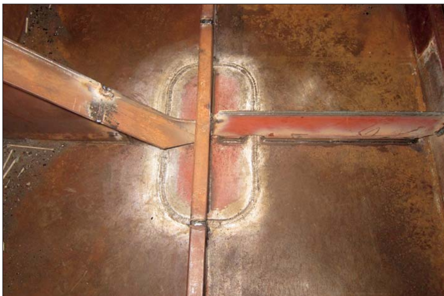
Fully welded insert plate with frames reinstalled.
