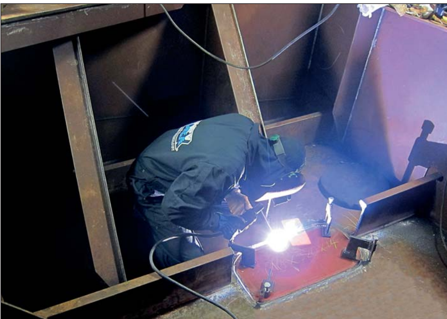
Certified welding securing a new insert plate.
