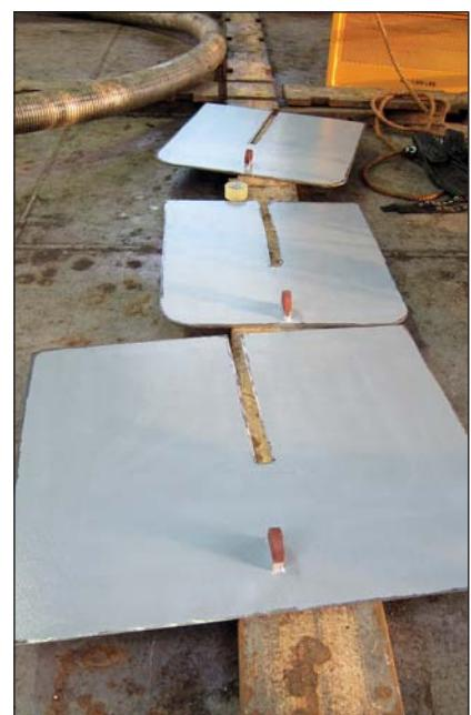
*Three of the doubler plates used to cover the damaged areas.*
