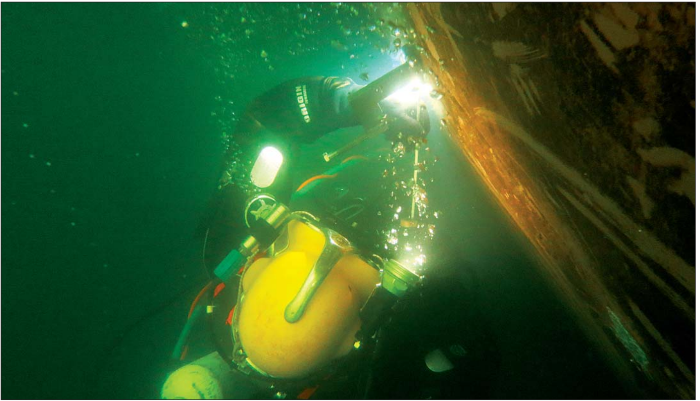
Diver/technician during welding work on one of the research vessels.
