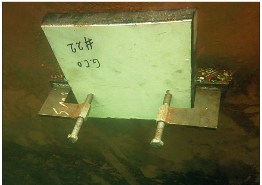
Blanks in a wide variety of shapes and sizes were installed on the four vessels.
