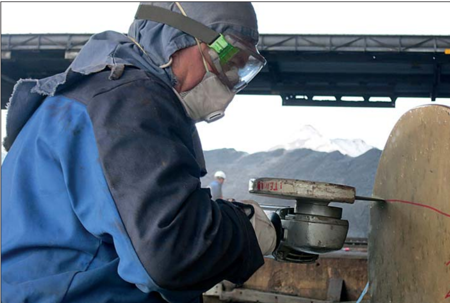
Modification of one of the blades of a bulker in Amsterdam.
