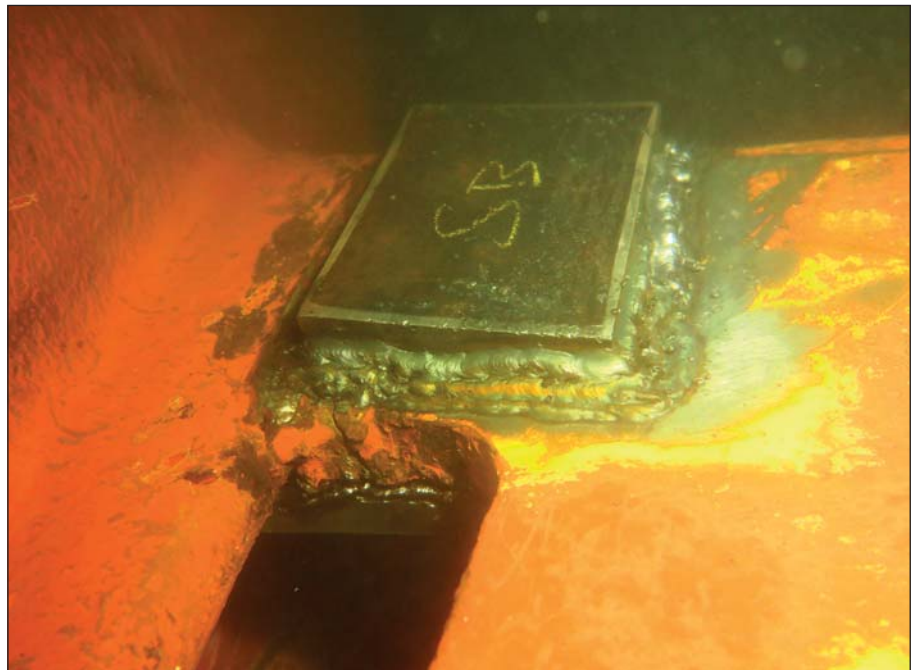
One plate was installed on the top of each crack and one on the bottom.
