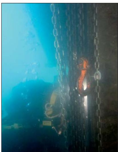
One of our divers performing welding work on the rudder.
