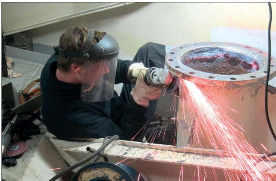
*Grinding out the corrosion on the outside of the pipe.*
