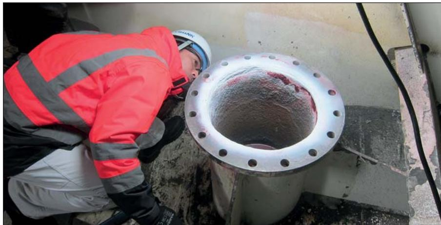
*Class surveyor inspecting the new weld seam.*
