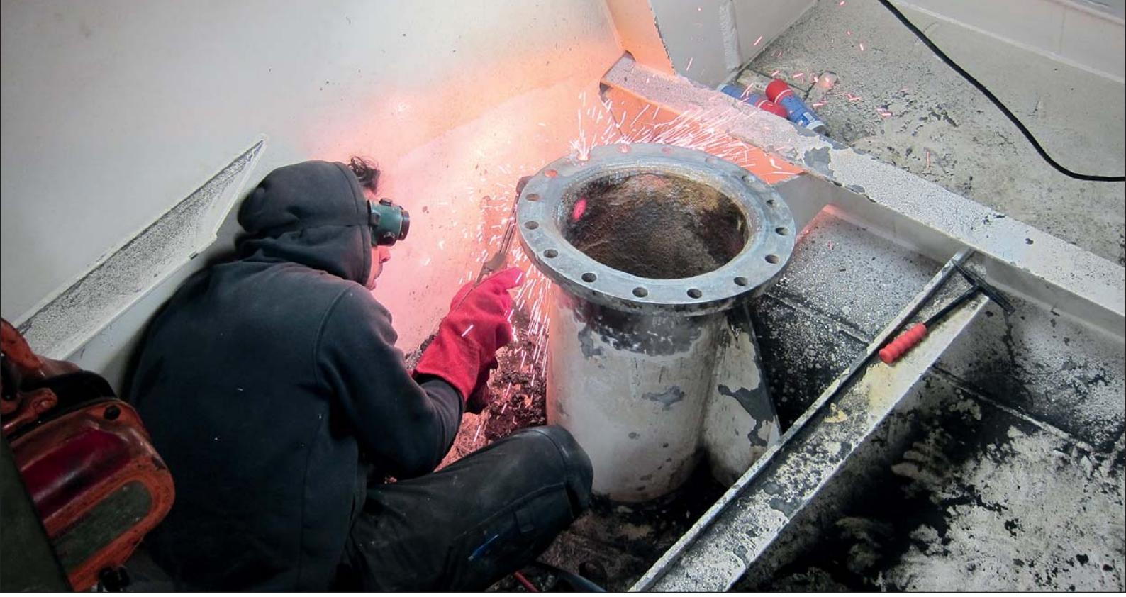
*Welding a new seam on the outside of the pipe.*
