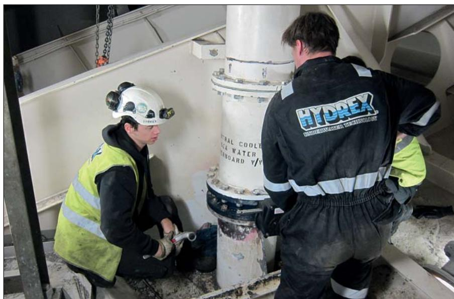
*Reinstalling the valve and the removed section of the pipe.*
