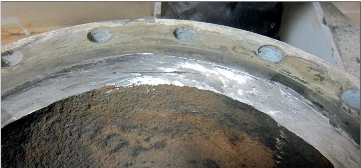
*Inside of pipe ready for new weld seam.*
