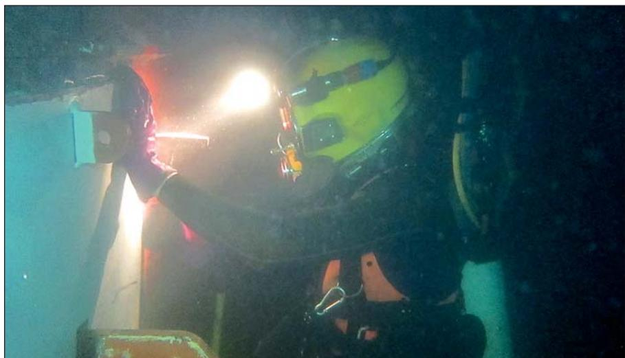
*Inspecting the welded doubler plate.*
