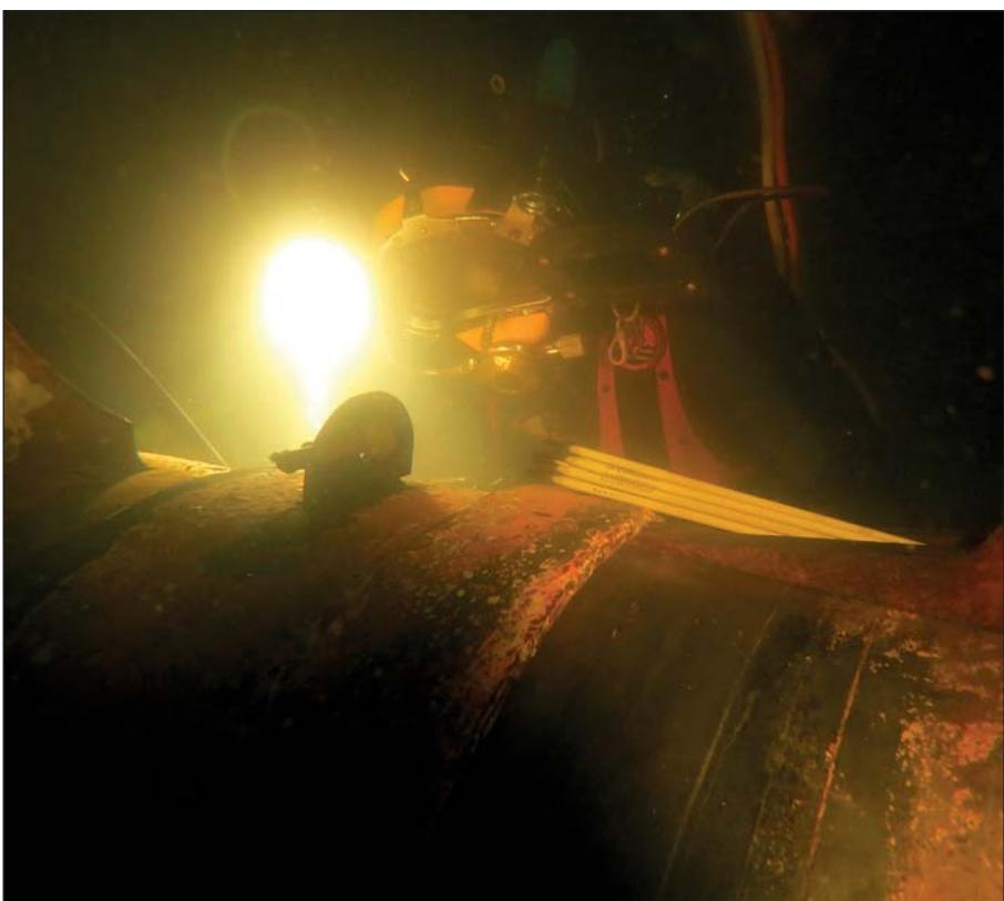
The rope guard was reinstalled after the successful seal replacement.
