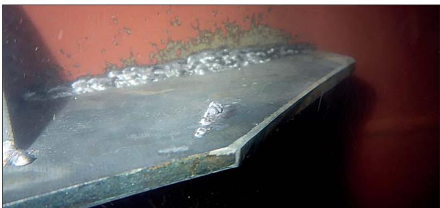
*A stiffener was installed over the doubler for extra protection.*
