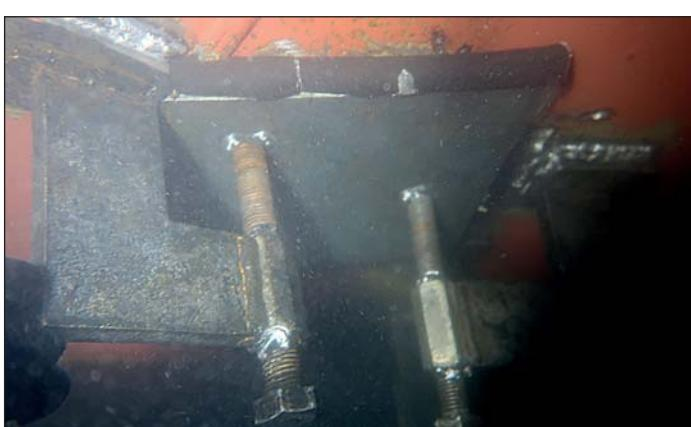
*Patches were installed over the smaller holes in the hull.*
