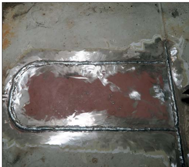
Insert after full penetration weld.
