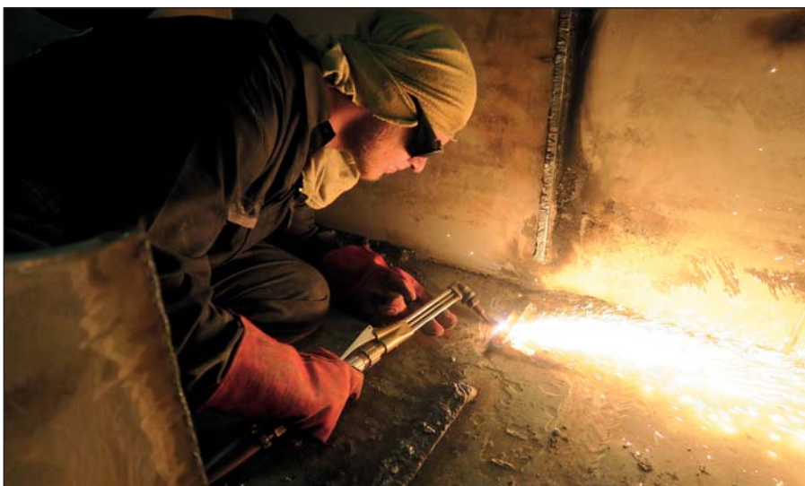
Removal of the damaged area.
