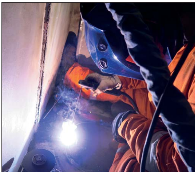
Welding the insert.
