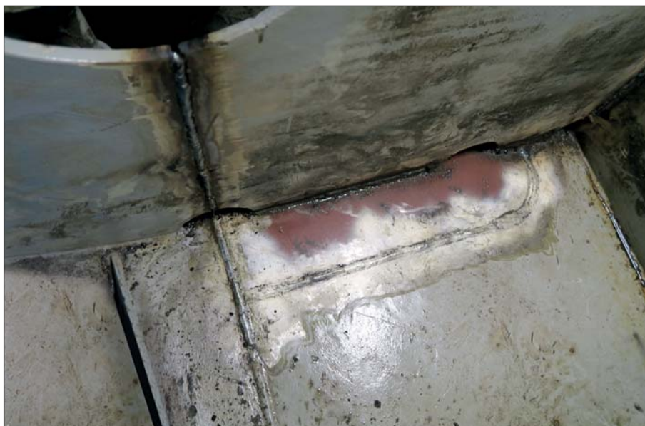
New insert after reinstallation of the frame covering the area.
