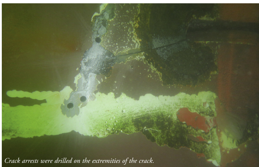
Branching crack on rudder of roro ship.
