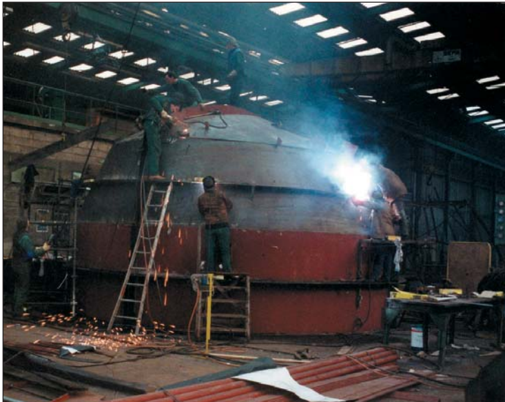
Constructing the replacement bulbous bow.
