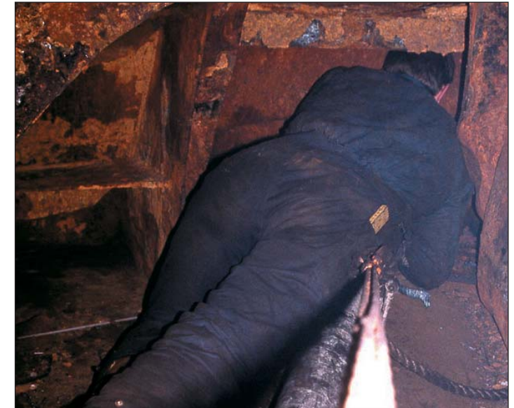
Additional reinforcement beams were welded into place.
