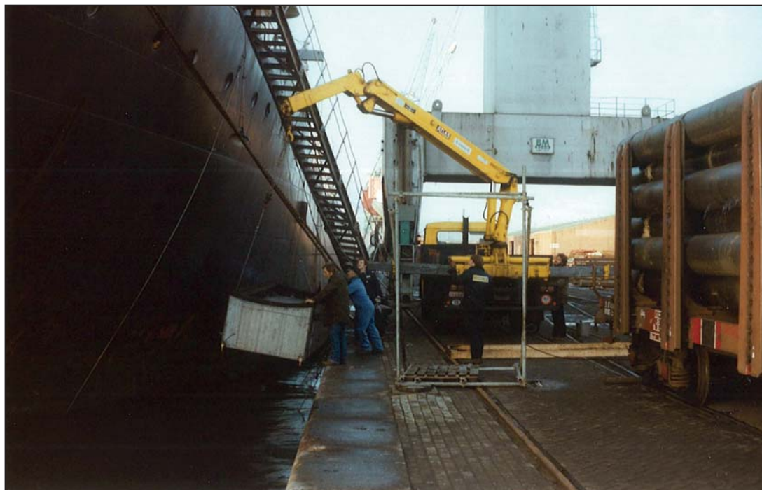
Lowering the cofferdam into the water.
