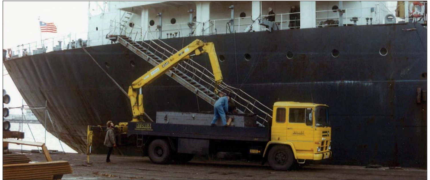
First prefabricated cofferdam ever used for afloat repairs arriving on-site, Antwerp 1979.
