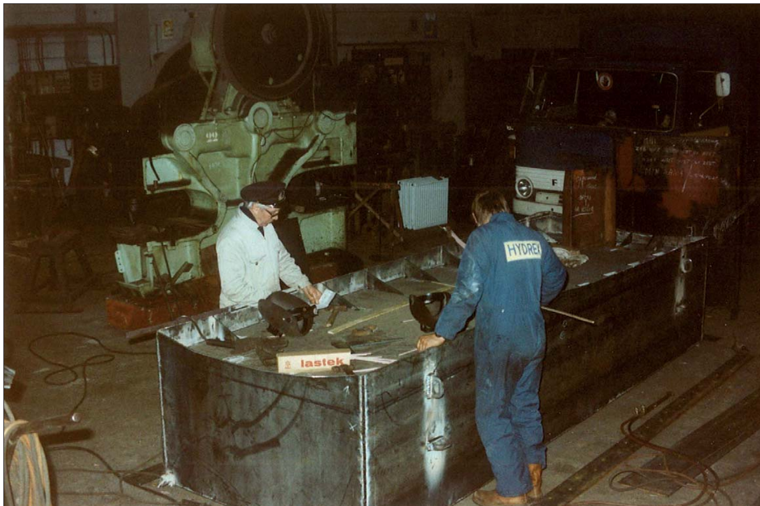
Construction of prefabricated cofferdam in our workshop.
