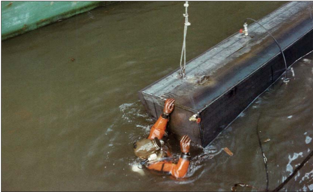
Hydrex diver guiding the cofferdam to its position.
