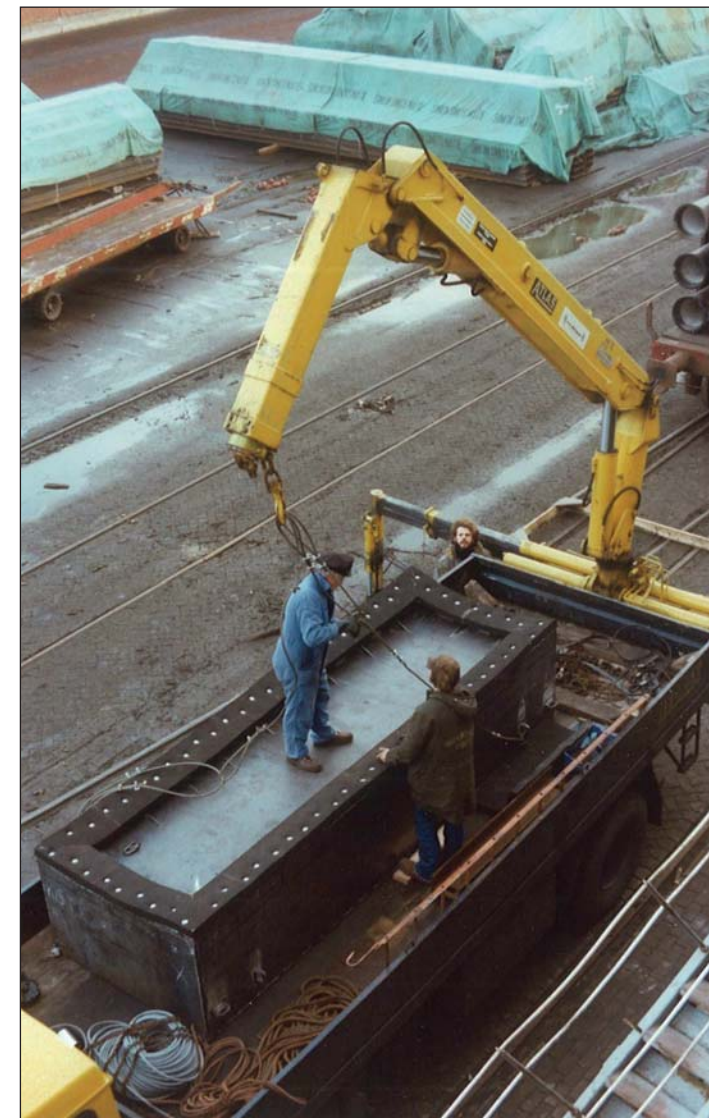
Arrival of the cofferdam on-site.
