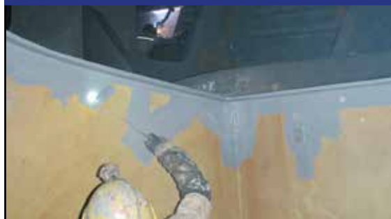
Applying RS500P with hot-work going on nearby
