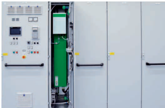
The ABB ACS 880 with active filter solution
