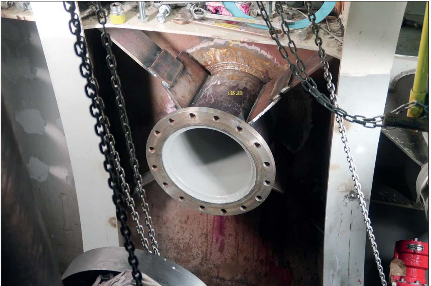
*New overboard scrubber pipe with Ecospeed protection on the inside.*
