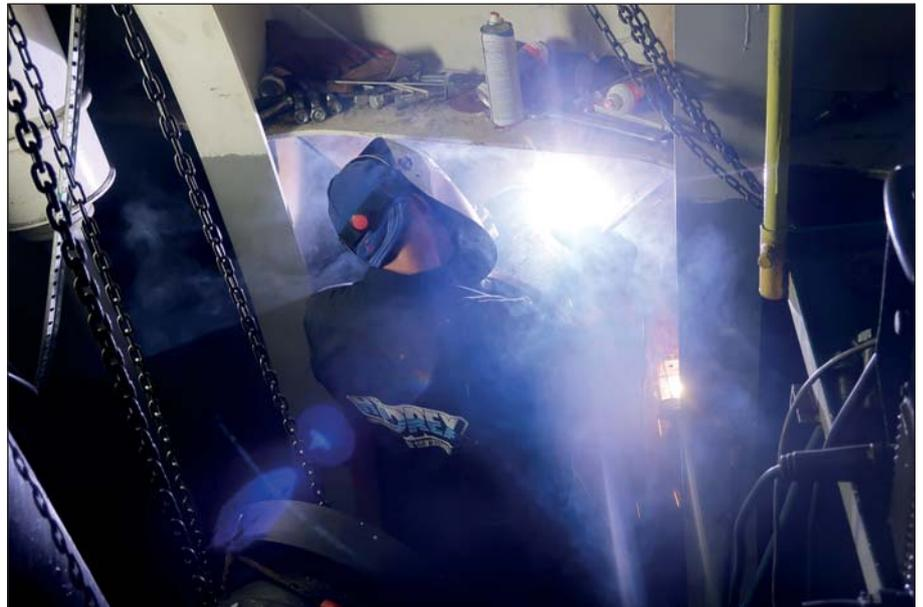
*Hydrex welder during installation of the new pipe on the bulker.*
