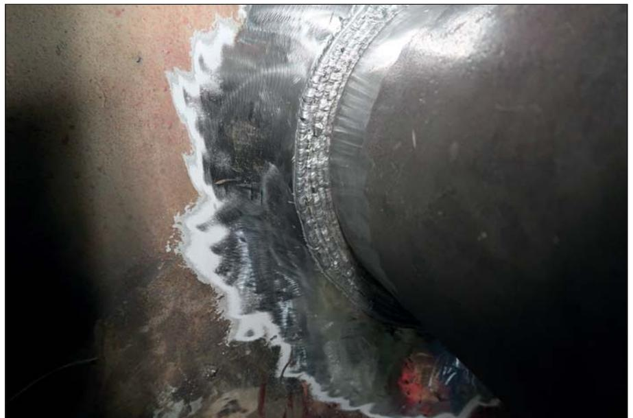
*The new pipe was secured with a full penetration weld.*
