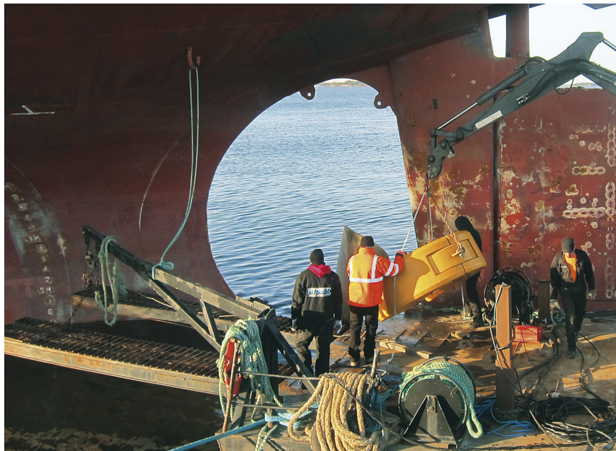
Diver/technicians positioning the latest version of the Hydrex cold straightening machine over a bent propeller blade
