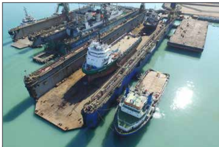
The ‘Namdock’ floating dock at EBHN
