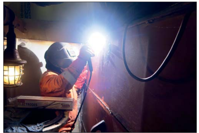
Securing the new inserts with full penetration weld.
