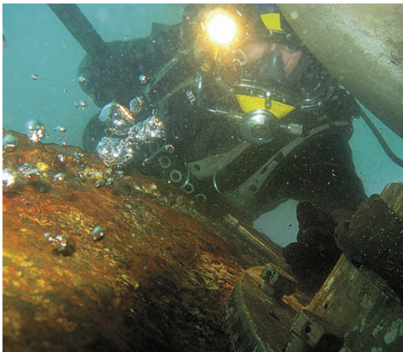
Diver working on a seal assembly
