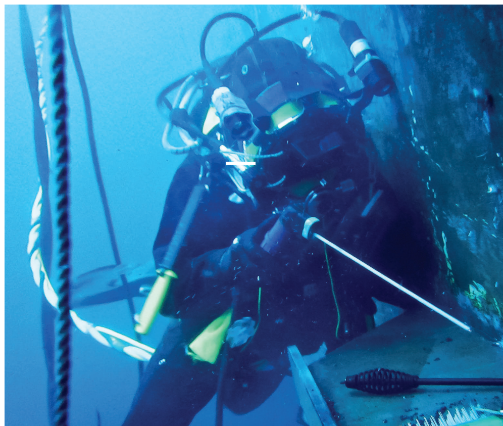
Fig. 13 — Strip welding the longitudinal stiffeners in place on the shell plate.
