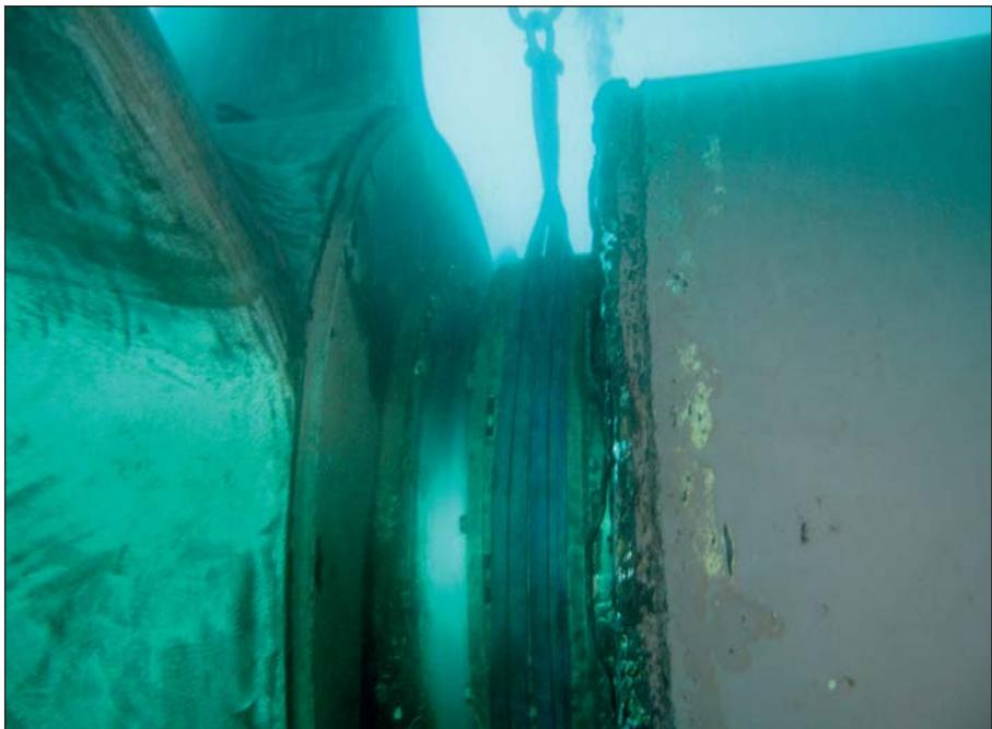
*Rigging the seal housing prior to installation of new gasket.*
