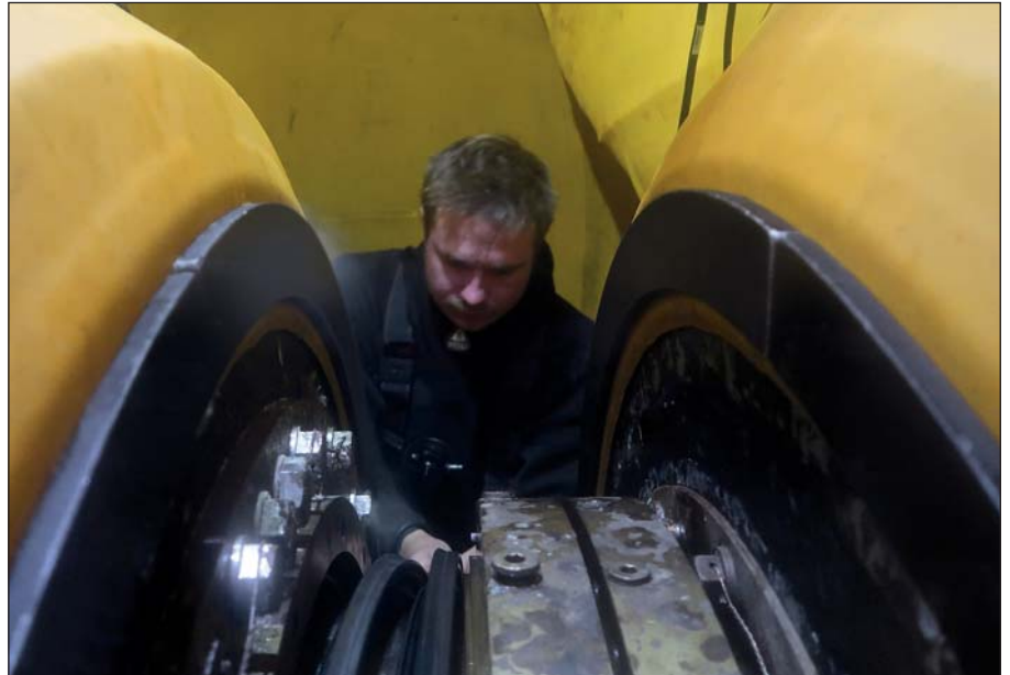
With our mobdocks we create a dry working environment underwater.
