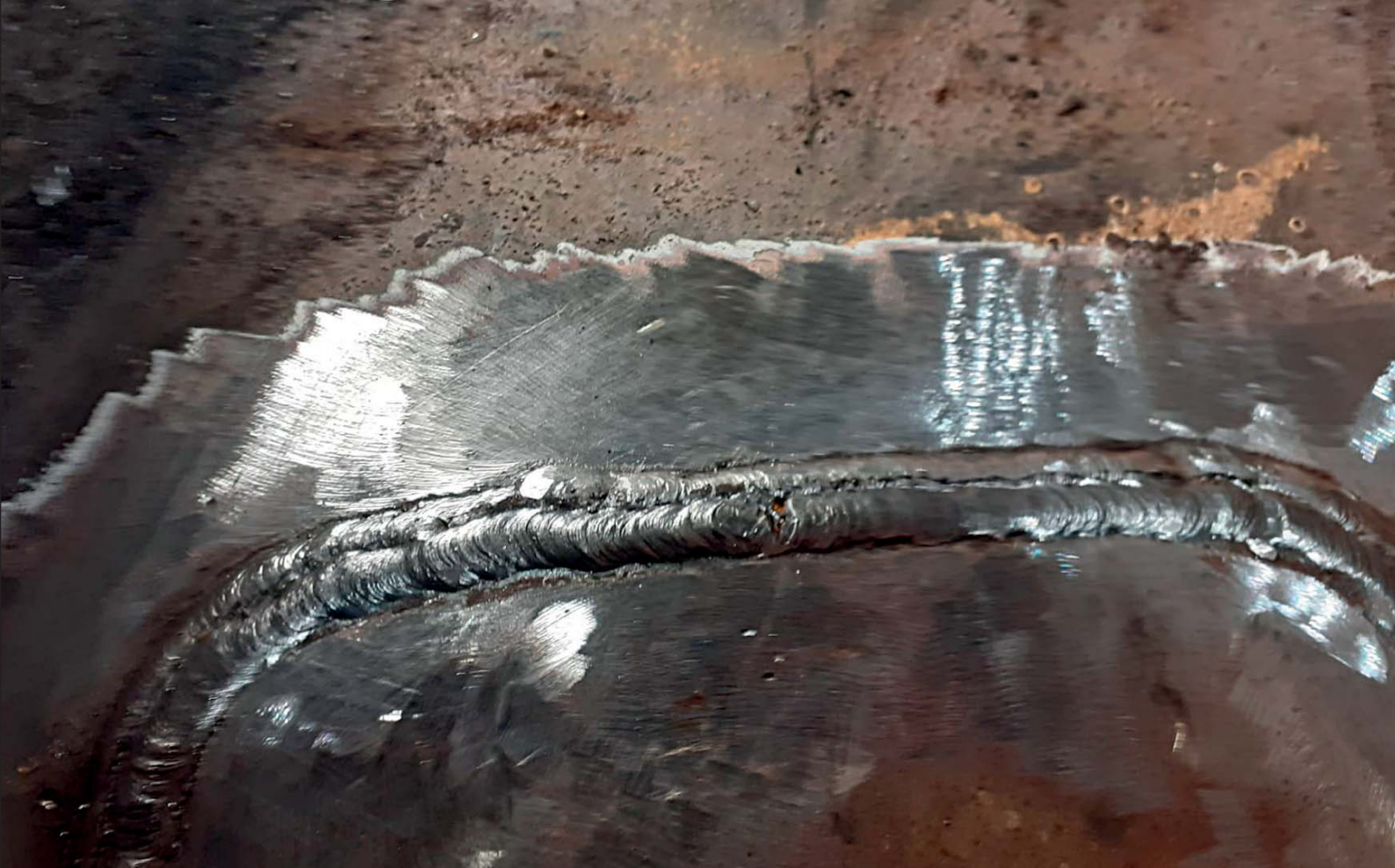
The insert was welded following our class-approved procedure.
