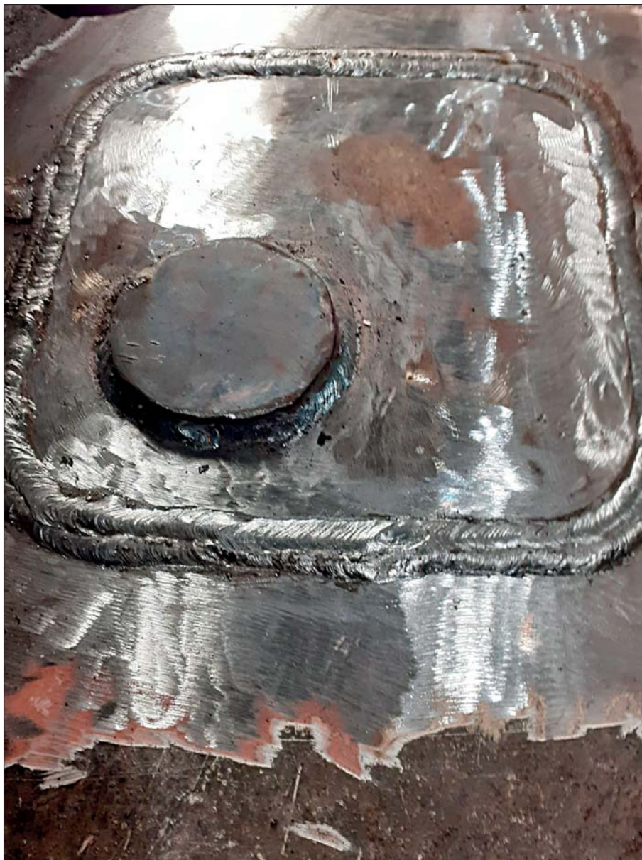
A small doubler plate was installed under the pipe to prevent the new insert from eroding again.
