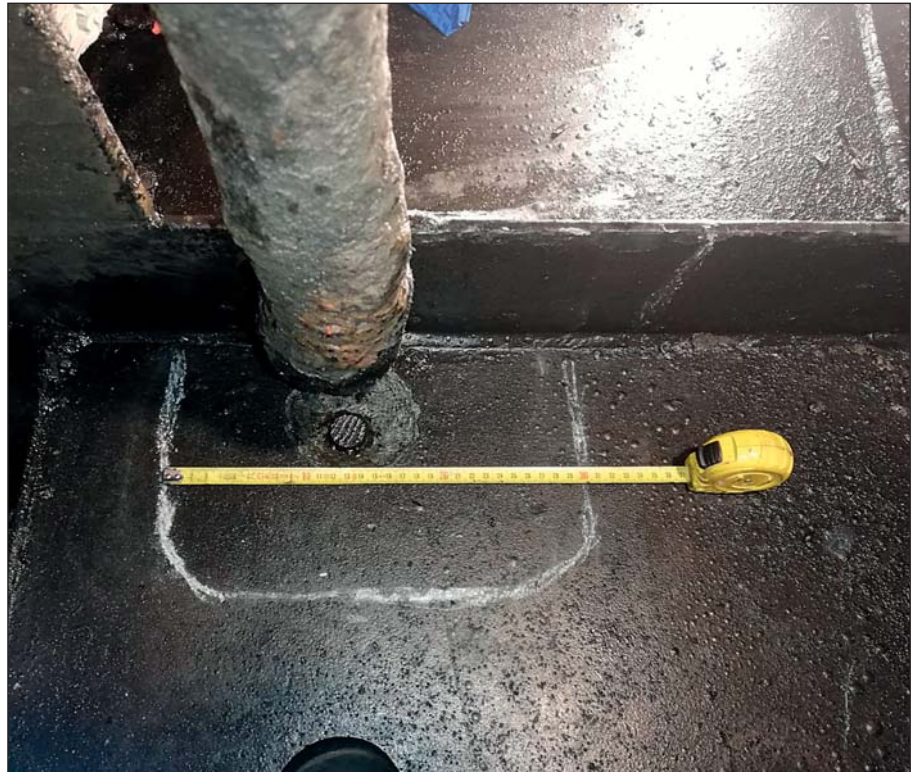
Measuring and marking the exact area that needed to be removed.
