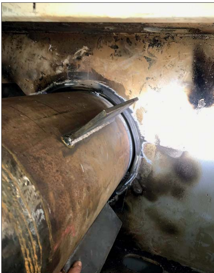
The new pipe was secured with a full penetration weld.
