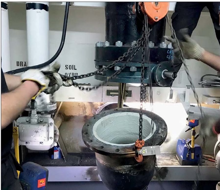
Positioning the new scrubber pipe on tanker.
