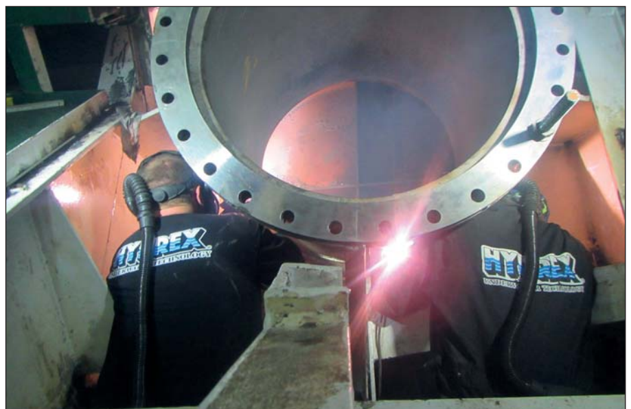
Our welders during installation of the new pipe on container vessel.
