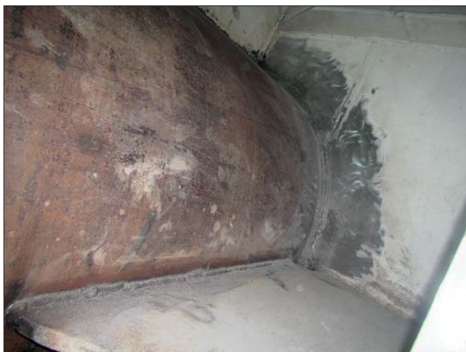
Scrubber pipe after welding and installation of the brackets.
