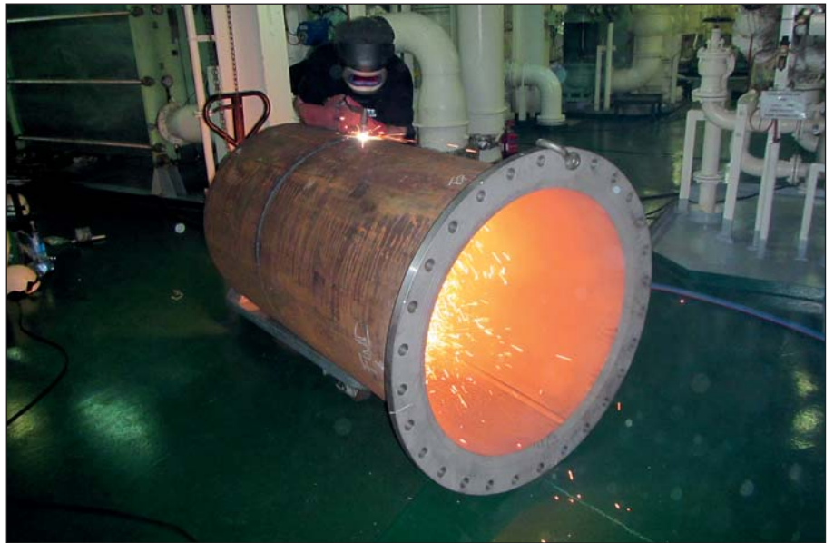
Preparing the new scrubber pipe for installation.
