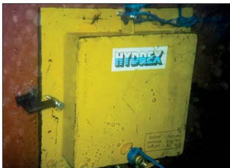
Cofferdam placed over crack.
