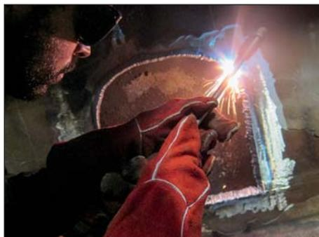
*Removing the damaged area.*
