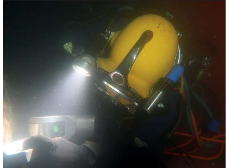
*Preparing the bow thruster for underwater removal.*
