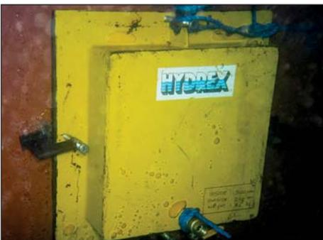
*Cofferdam placed over crack.*
