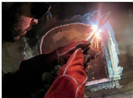
Removing the damaged area.
