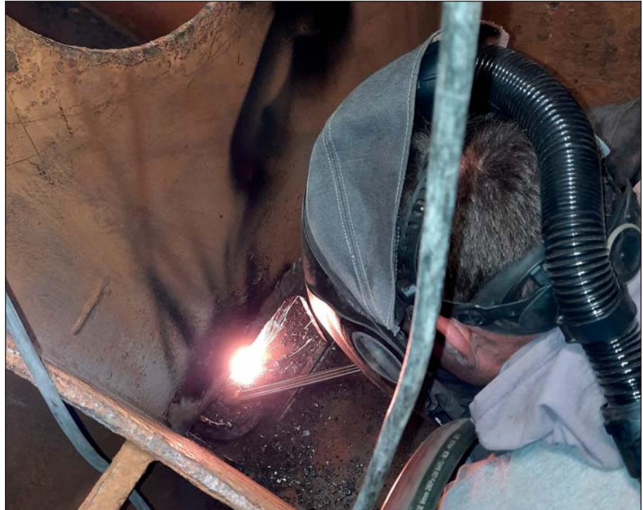
*Removing damaged shell plating on tanker in Rotterdam.*
