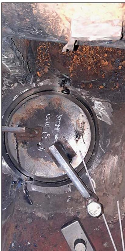
*New insert positioned and ready for welding.*
