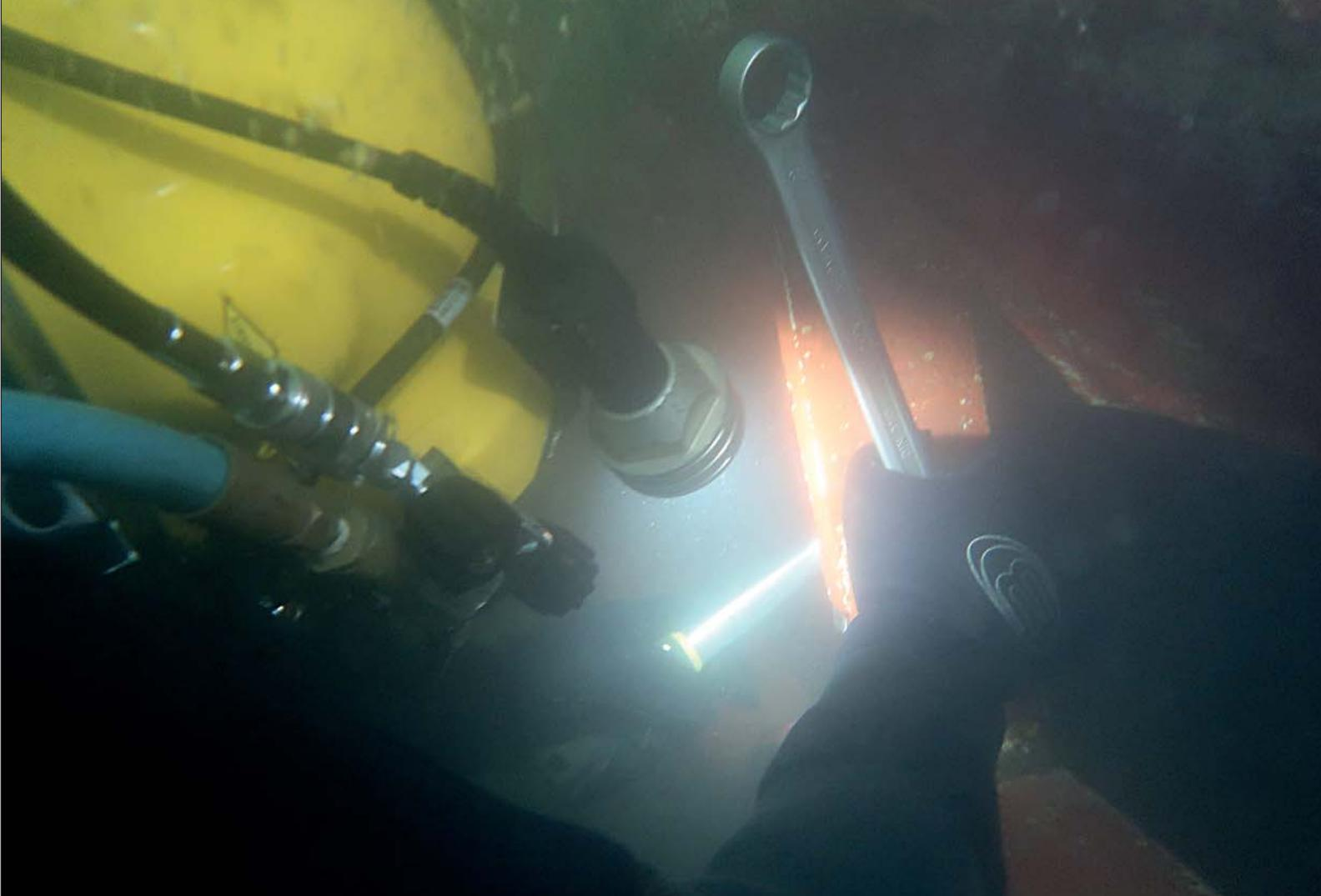
*One of our divers reinstalling thruster tunnel grid bolts.*
