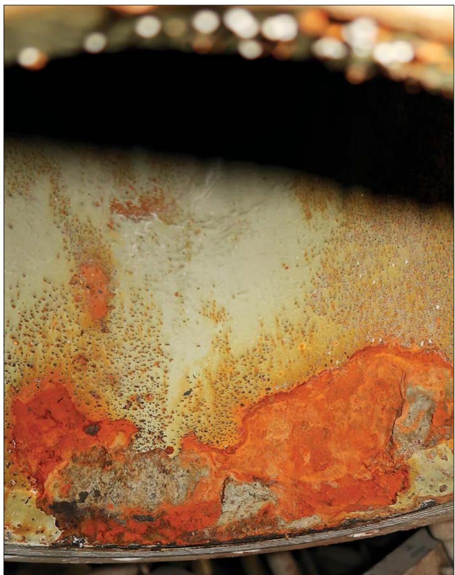
Corroded scrubber pipes on bulker.
