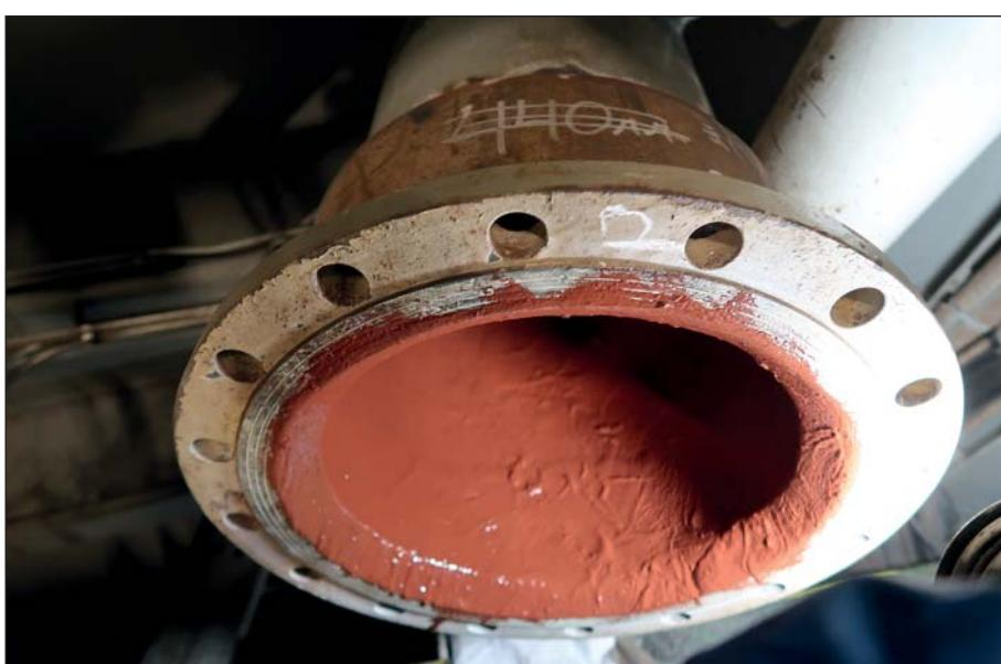
Inside of pipe coated with Ecospeed to prevent further corrosion.
