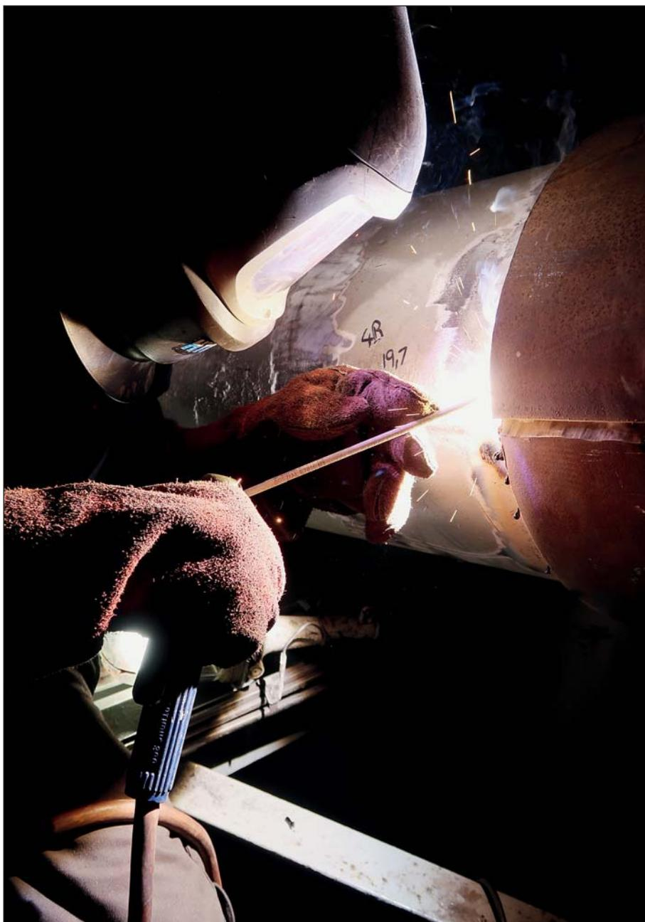
Hydrex welder installing reinforcement shell.
