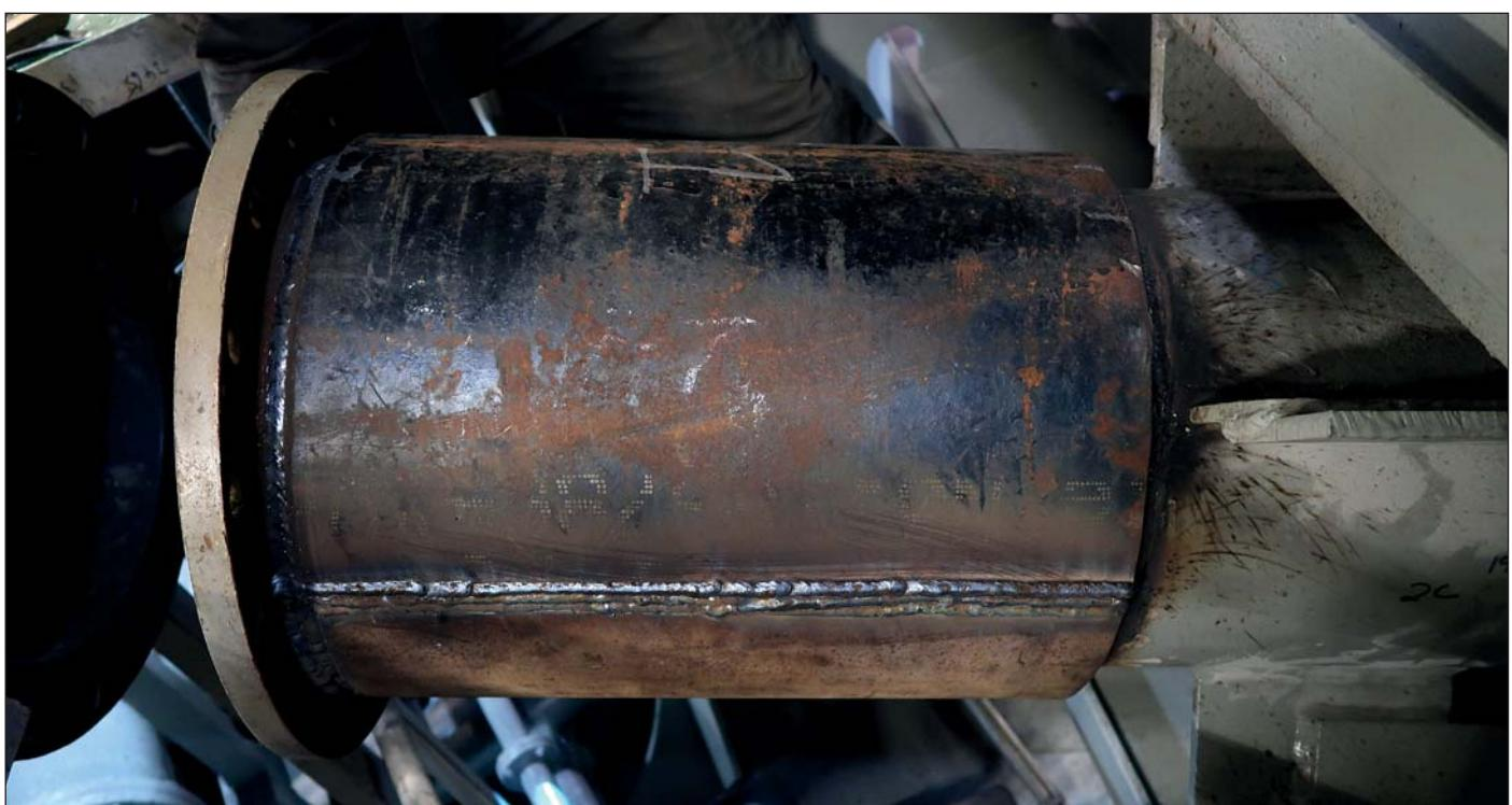
*Reinforcement shell around overboard pipe.*
