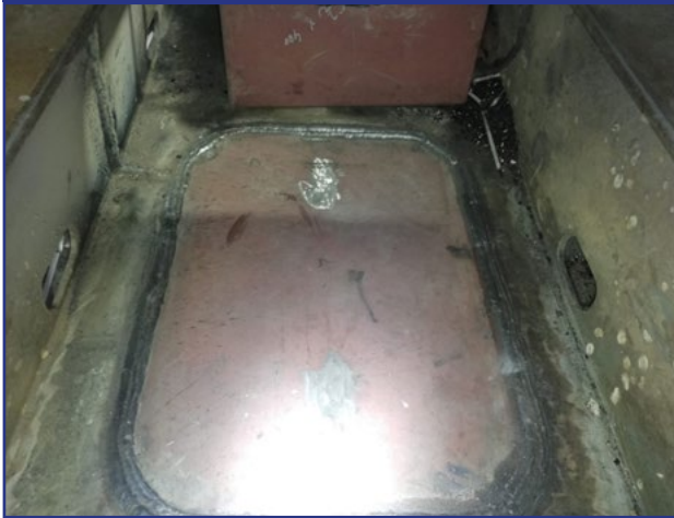
The new insert installed on the containership
