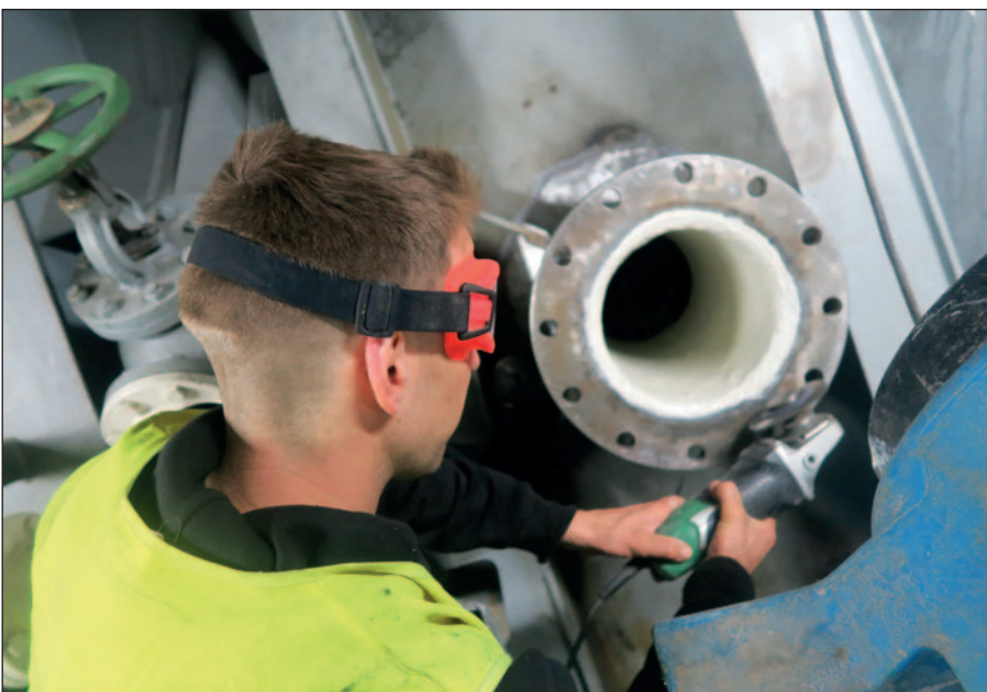
Final work on the flange of the new scrubber pipe in Antwerp.
