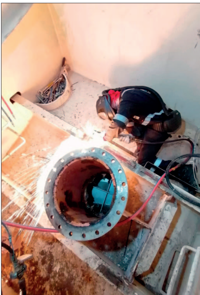
Hydrex diver/welder during installation of a new scrubber pipe.
