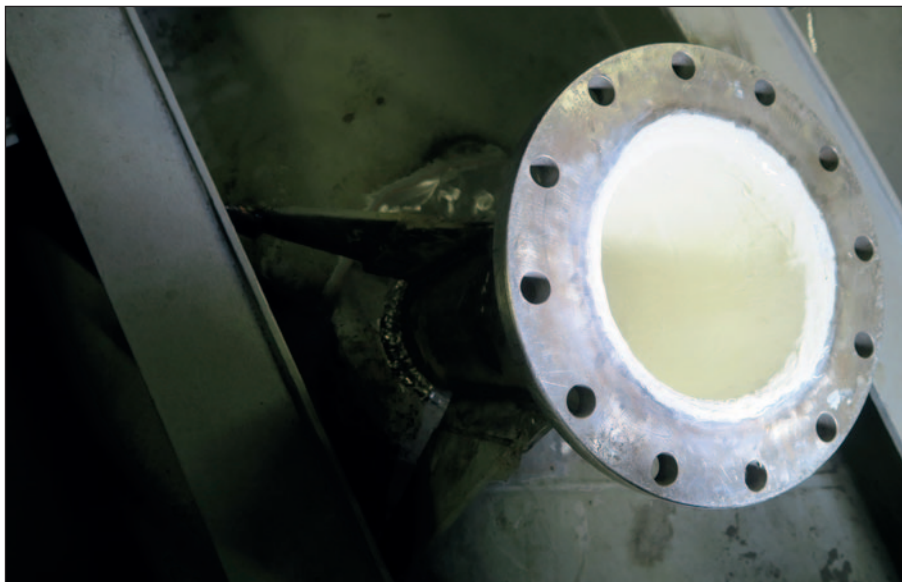
New scrubber pipe coated with Ecospeed.
