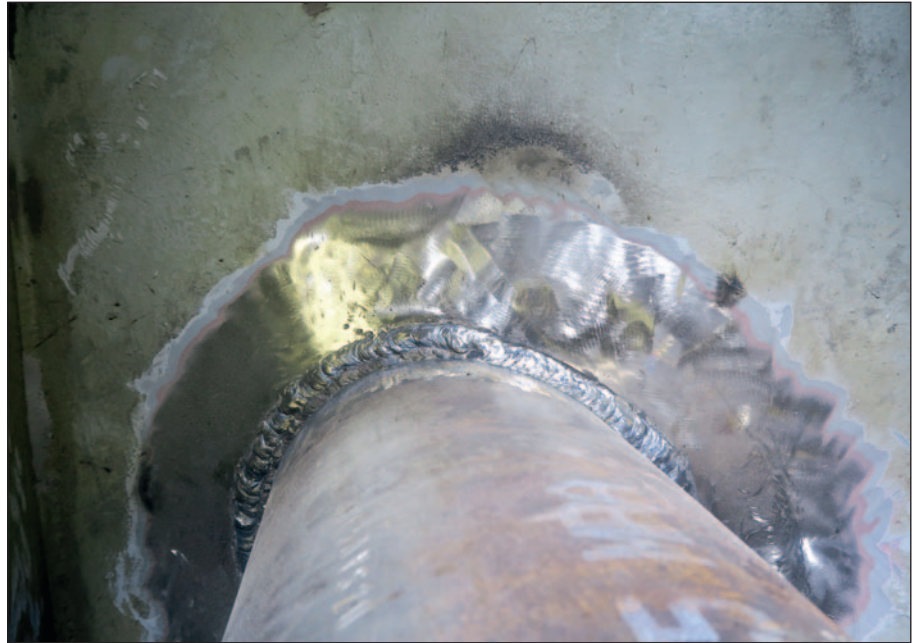
New scrubber pipe on tanker after welding.
