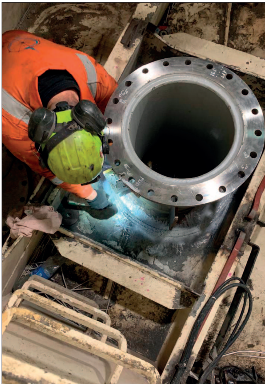
Independent inspector checking the welds.
