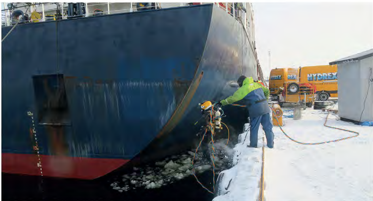
A HYDREX DIVER BRAVING HARSH WEATHER CONDITIONS TO CARRY OUT PROPELLER STRAIGHTENING
