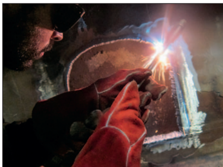
Removing the damaged area.
