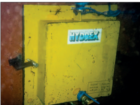
Cofferdam placed over crack.
