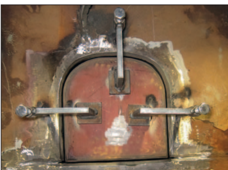
Insert cut and fitted.
