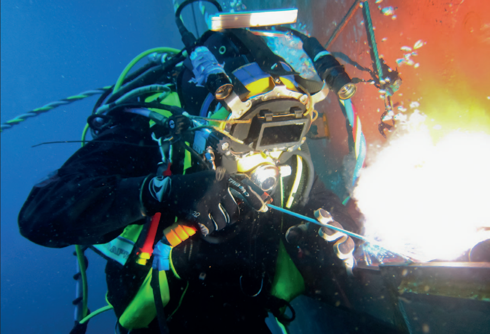
Underwater welding by a well-trained and properly-equipped Hydrex diver.
