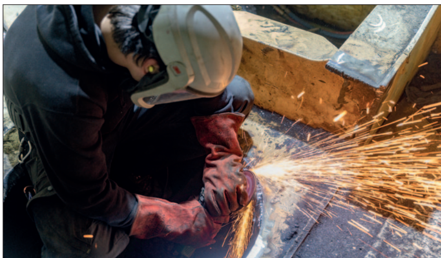
Safety is just as important during dry work inside the ship as under the water when diving. Here, one of our Third Divers grinds a bevel on the hull of a ship prior to a full penetration weld to install a scrubber outlet pipe.
