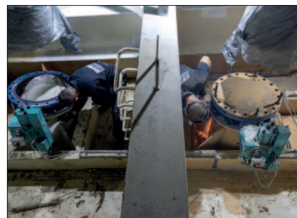
Routine scrubber overboard installation
