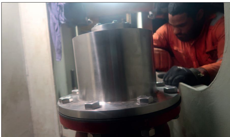
After the NDT test the valve was installed on top of the flange.
