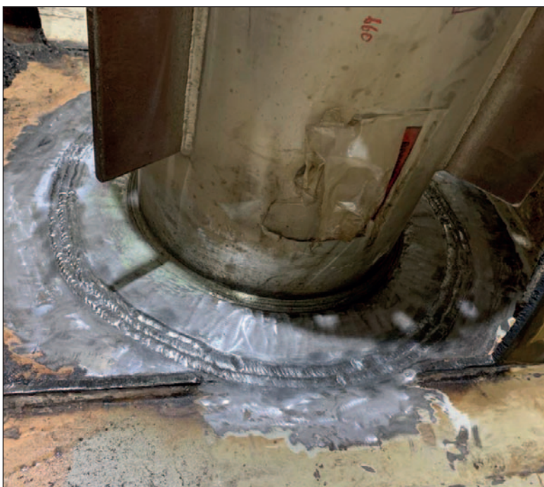
Multipass, multilayer full penetration weld attaches the new pipe to the hull.
