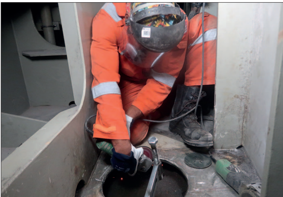
Preparing the edges of the hole.
