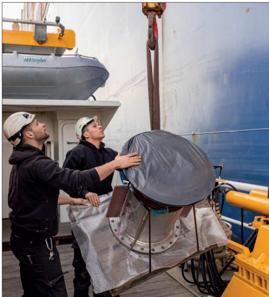
The replacement scrubber overboard pipes are hoisted up to the ship to be taken to the engine room.
