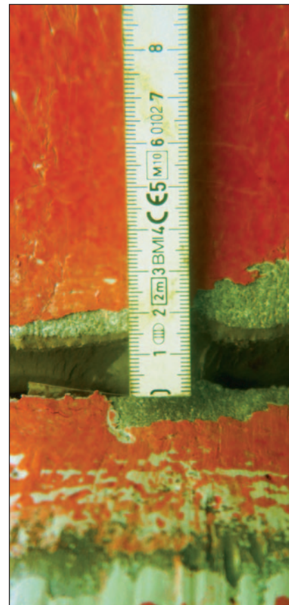
Measuring the width of the crack.
