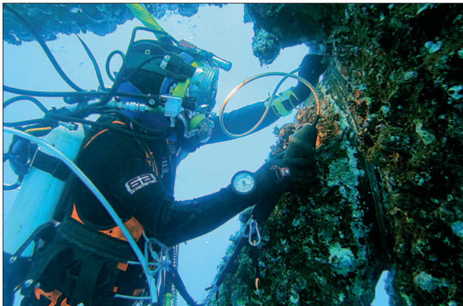
Diver inspecting a heavily fouled offshore structure.
