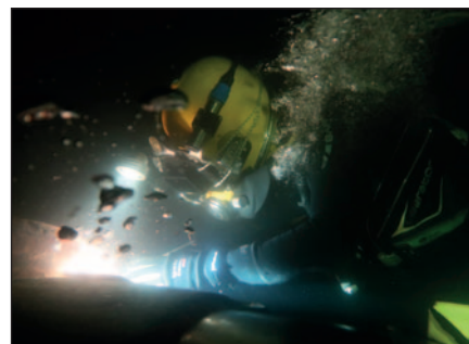
Underwater repair of leaking seal assembly in Trinidad 4-7
