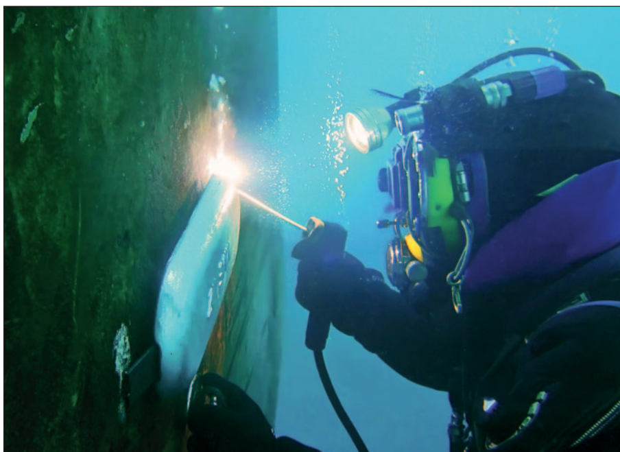
Anode replacement is a relatively straightforward operation to perform underwater without the need for drydocking.
